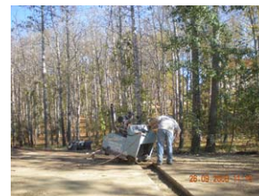
Concrete/Asphalt Cutting
